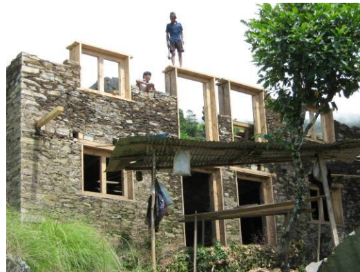
New building under construction (October 2008)
