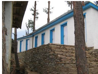
Toilet block - two far toilets are the original teachers' toilets.
